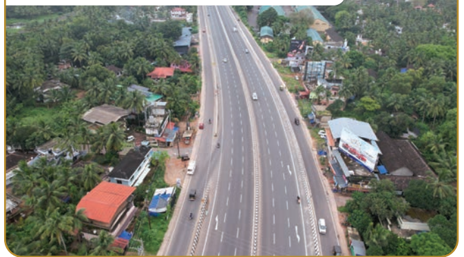
Aerial View of the completed highway
