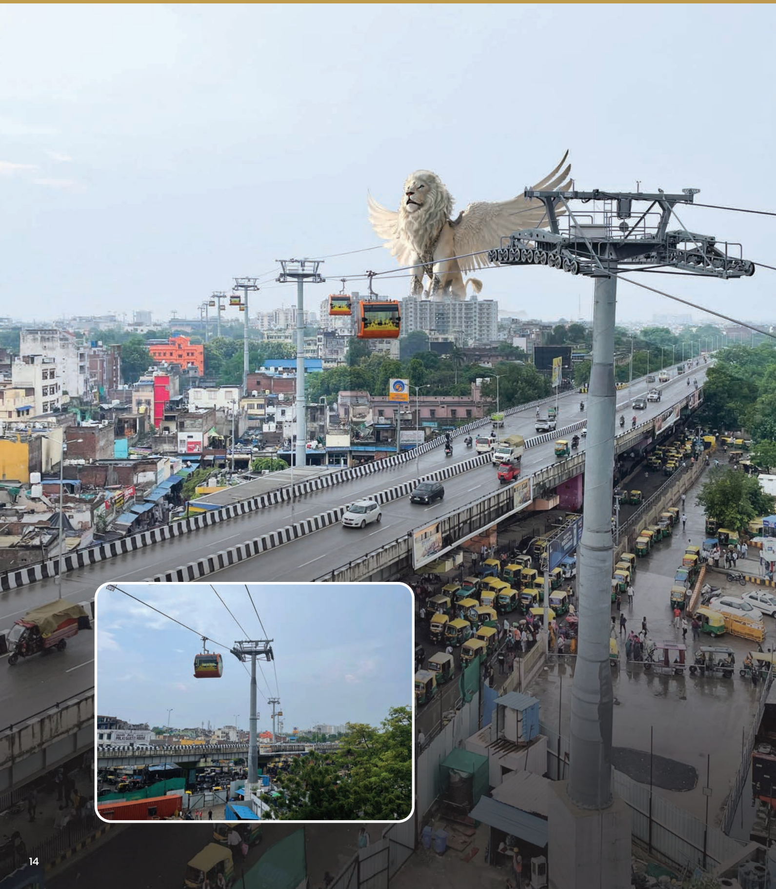
Testing of the Varanasi Ropeway Project in progress.
