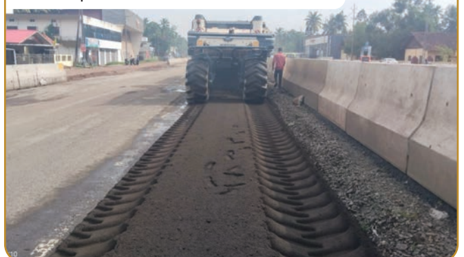
FDR in process with StabilRoad
